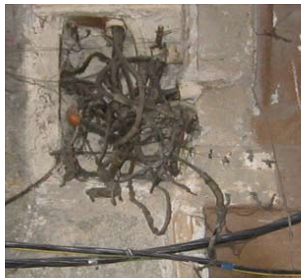
An example of electric mains in which KYP Alliance has exploited a PLC channel
